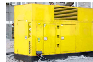
発電機 [筐体内張り吸音材・断熱材 (耐熱性)] Power generator [sound-absorbing material attached inside the housing, heat insulation material (heat resistant)]
